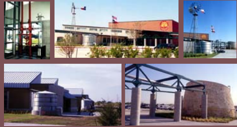
Roy Lee Walker Elementary, McKinney, TX
