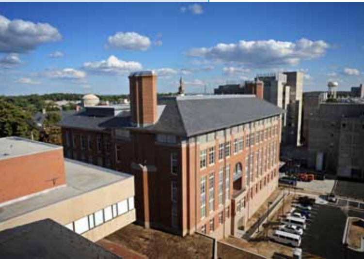
The Carolina Physical Science Complex is the most ambitious construction project in the University's history.
